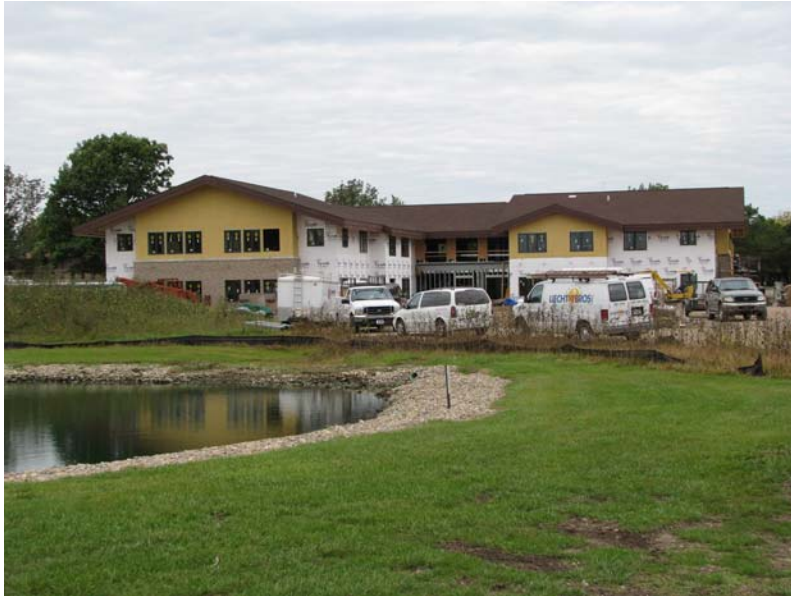
Swiss Village East Wing Expansion Project.
